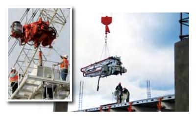
Four pin quick-disconnect and quick-release hydraulics allow the boom to be flown and mounted in a matter of minutes including from truck-mounted pumps with optional detachable booms. Hydraulic powerpack (left) can be flown separately to reduce picking weight.
