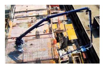
Schwing's four-section Roll & Fold<sup>TM</sup> boom design combines 694 degrees of usable boom articulation allowing operators to place concrete back to the mast at any elevation and cover thousands of square feet from one location.
