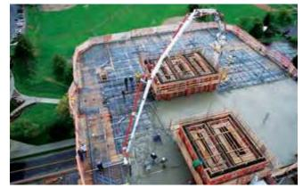
With 730-degrees of rotation, the separate placing boom efficiently places all your elevated concrete.
