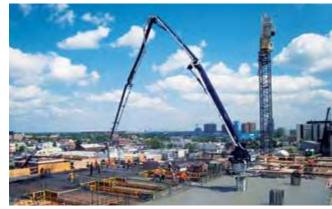
Wireless proportional boom controls provide precision placement without interference from other competing signals. Integrated hydraulic power pack is operated off of 460-volt electric motor.
