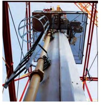
The galvanized expanded metal work platform provides worker stability for mounting the separate placing boom, routine maintenance and operation. Pipeline and ladder brackets are integrated in the design of every modular section allowing fast assembly. Lengthen the octagonal mast by adding 4 or 6-meter modular sections to accommodate the job, and simply add more ladder and pipe sections as required. Mast sections are quickly & easily joined together with 16 bolts.
